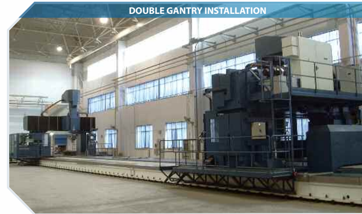
DOUBLE GANTRY INSTALLATION
